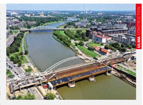
**Trusses**, 24 - 30 metres in length. This truss system is modular, requires minimal shoring, and is easy to assemble and handle. The narrowest span is made of 12 m long TAC steel profiles.
